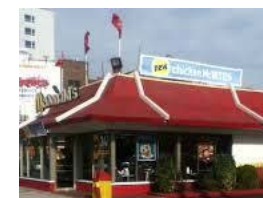
Roof mounted signs
